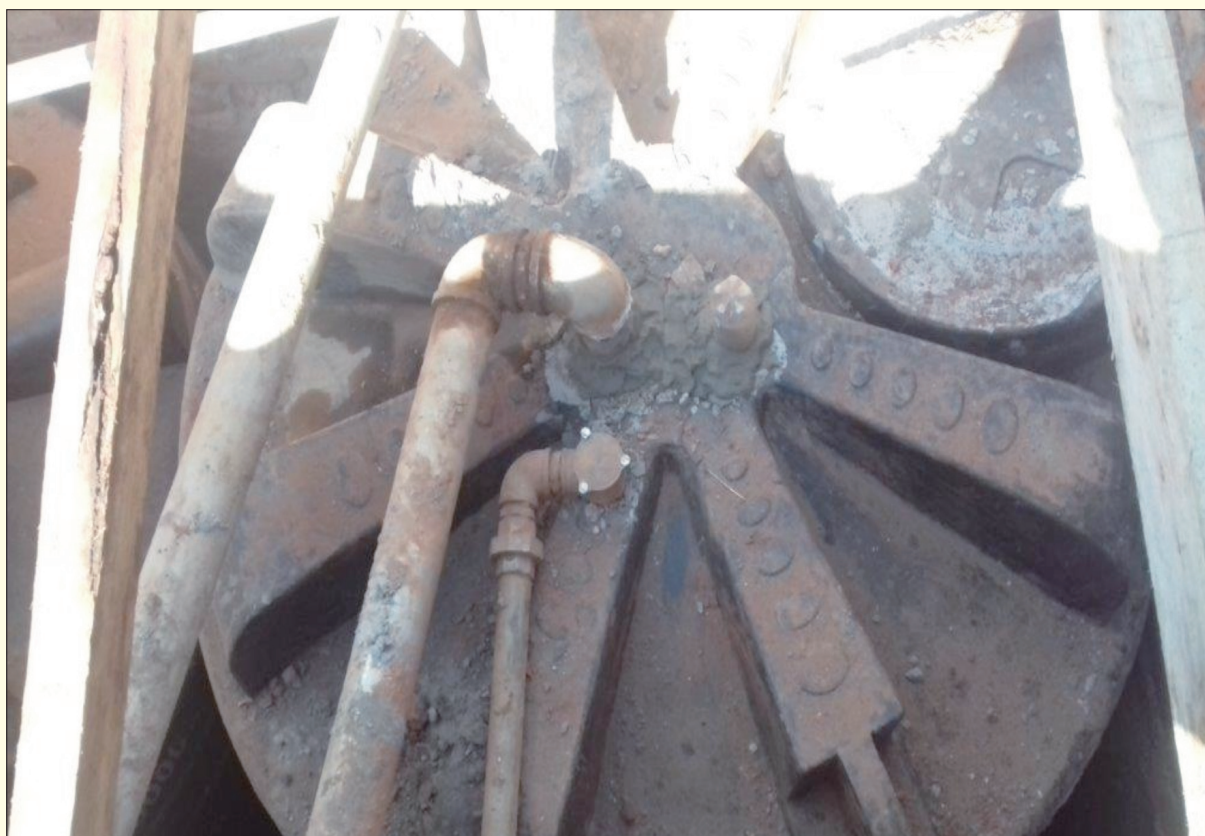
Figure 19: A sim tank which was being used by Manamba Lubricants Family to as an underground storage tank - Ludewa.
