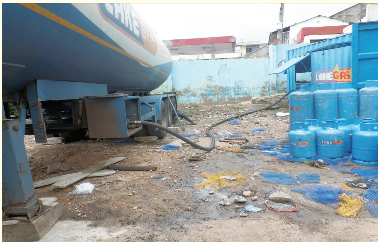
Figure 17: A hose pipe connected from the LPG storage facility to the filling point at Lake Gas Ltd – Kenyatta Road LPG Filling Plant in Mwanza.
